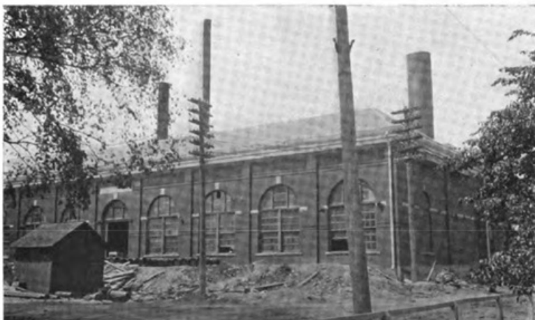
POWER STATION AT FINDLAY, TOLEDO URBAN & INTERURBAN
