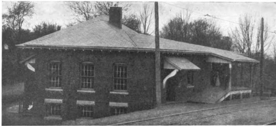
TYPICAL SUB-STATION, STARK ELECTRIC RAILWAY
