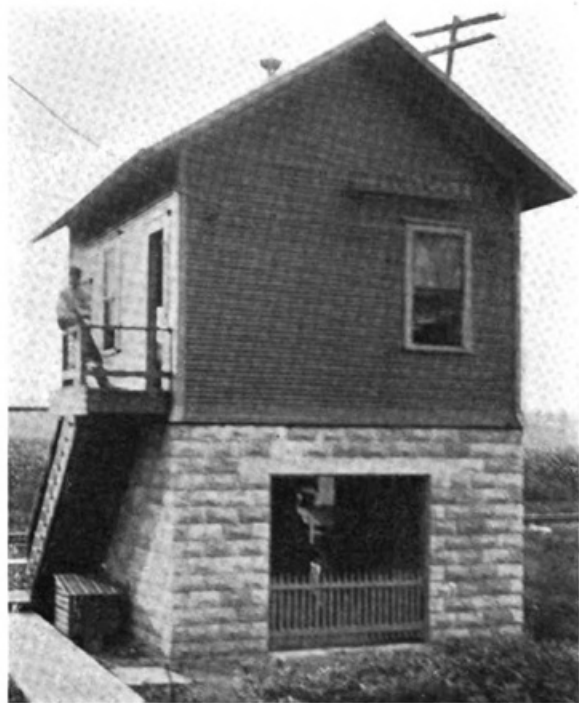
COMBINATION SWITCH TOWER AND SUB-STATION, TOLEDO & WESTERN
