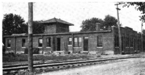
SUB-STATION AND BATTERY HOUSE, DAYTON & MUNCIE
