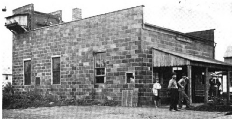
TILE SUB-STATION AND WAITING ROOM, CANTON-AKRON RAILWAY
