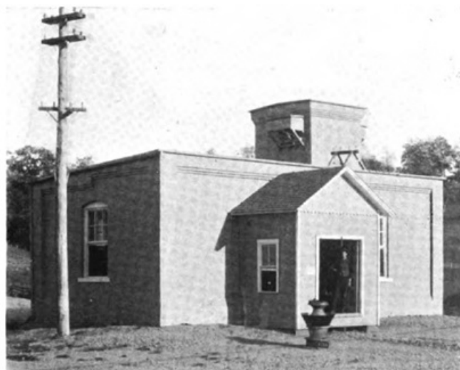
SUB-STATION, COLUMBUS, NEWARK & ZANESVILLE
