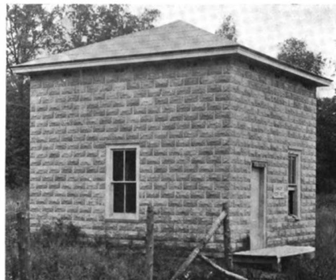
CONCRETE BLOCK SUB-STATION, TOLEDO & INDIANA
