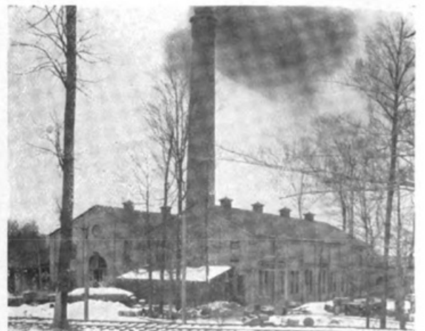
POWER STATION AT ELYRIA, CLEVELAND & SOUTHWESTERN
